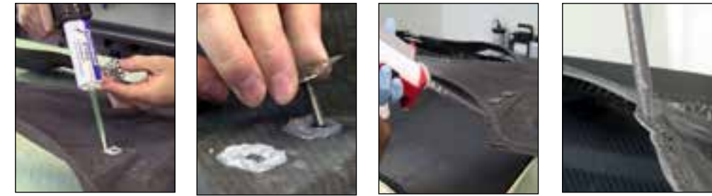
Permabond two part epoxy is used to bond fasteners to a carbon fiber car hood and Permabond PT326 bonds the 2 skins of a carbon fiber car hood together.
